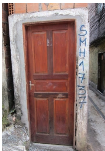
Figure 9. House marked for demolition, Providência, 2011 (Photo: A-M. Broudehoux)
